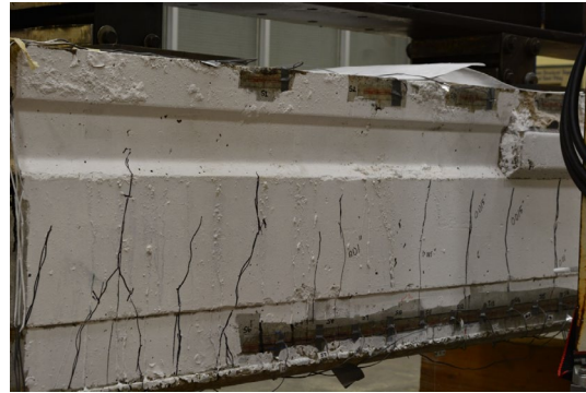
2. Induce Initial cracks
